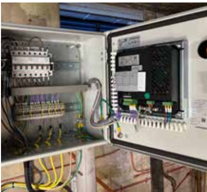
Inspecting sensor terminations and BMS connections
