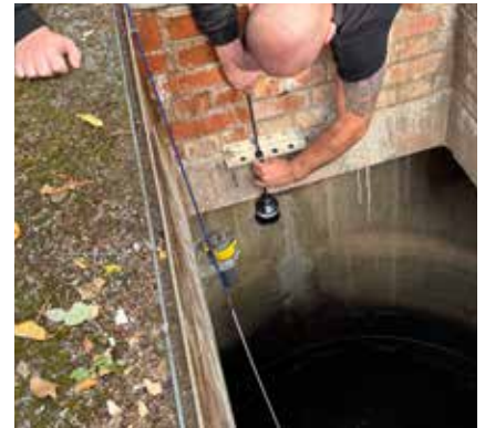
Installation of the new level sensor
