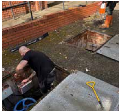
Pushing the electrical cable through ready for connection
