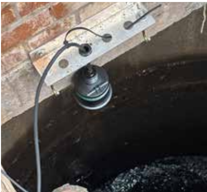
Ultrasonic level sensor installed and set at the correct height
