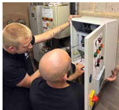
Installation of the new Pulsar control panel
