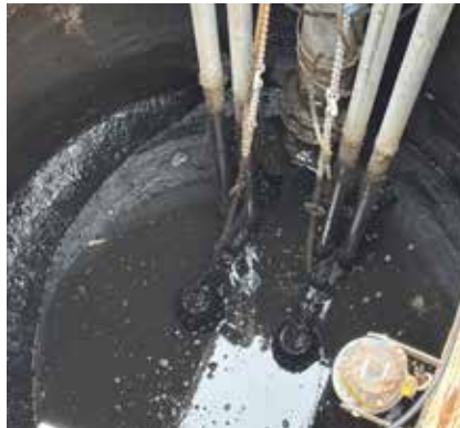
The two submersible pumps at the bottom of the wet well
