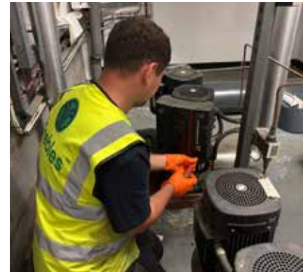
Disassembling the pump
