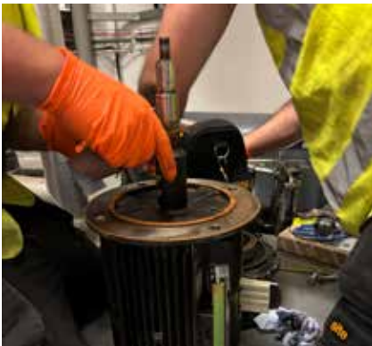
Inspection of stub shaft
