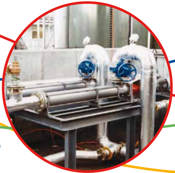
Pumping of slurry mix
